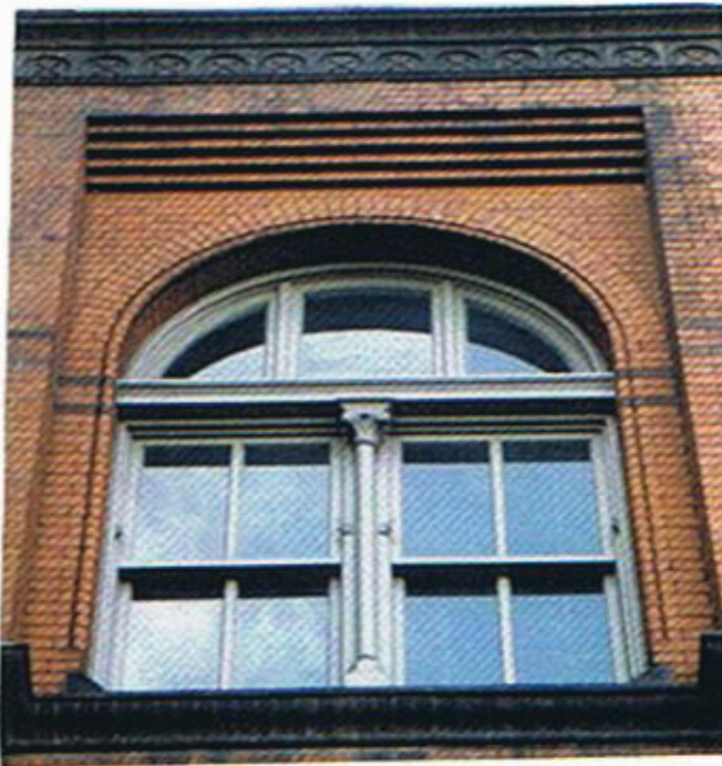
THE AUDITORS BUILDING LOCATION: 14TH AND INDEPENDENCE AVE, WASHINGTON DC DATE: April 86 - Feb. 87 CONTRACTOR: Camden Millwork Inc., NJ SCOPE: Restore 960 window frames and replicate sash using 1/2 IG glass.
